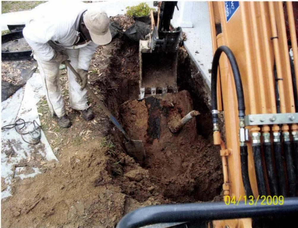
Picture 2: UST 274Birch during removal from excavation.
